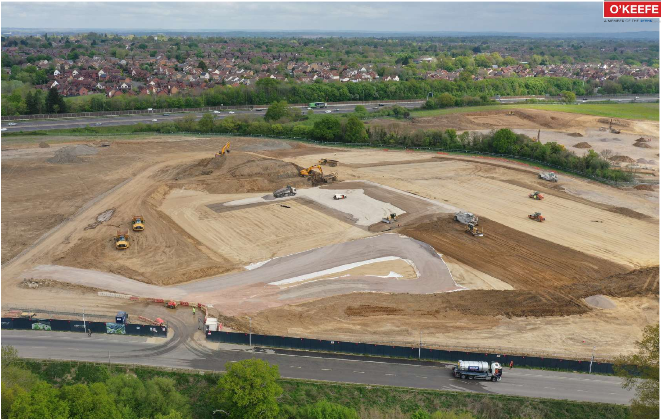
Disney Studios, Shinfield | Curo Construction | 50 Weeks | £7.0m
