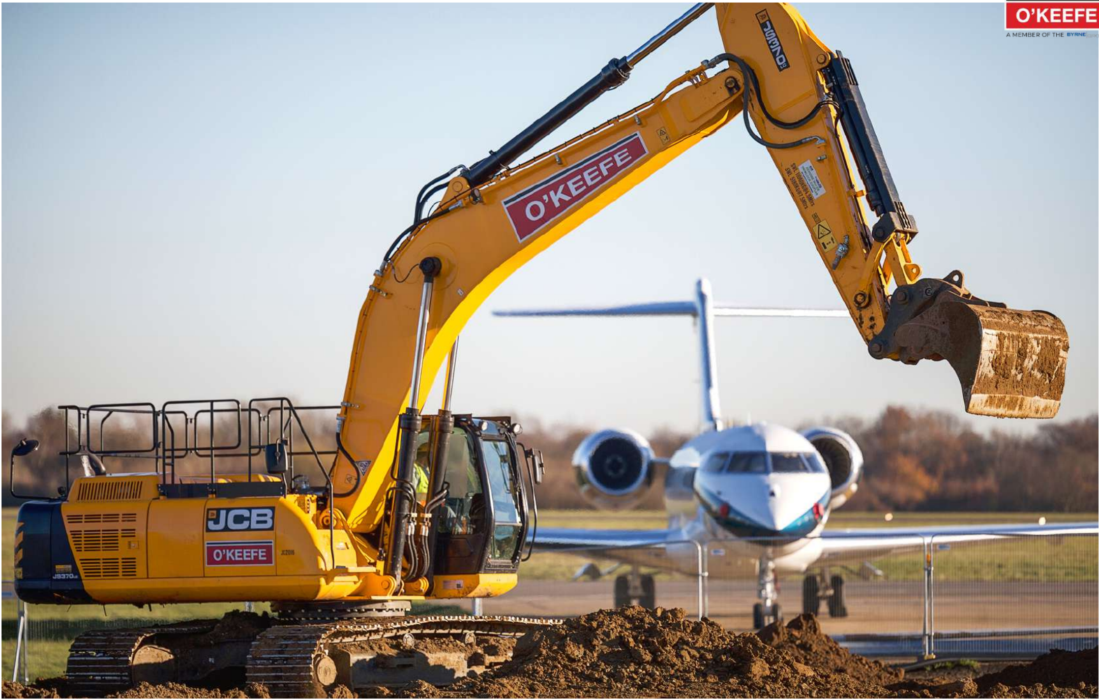
Biggin Hill Airport | Civils Construction | 44 Weeks | £1.5m
