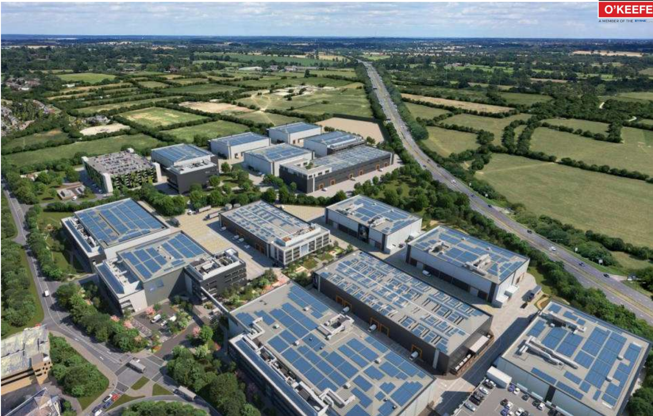
Sky Studios, Elstree | BAM Construction | 20 Weeks | £1.8m
