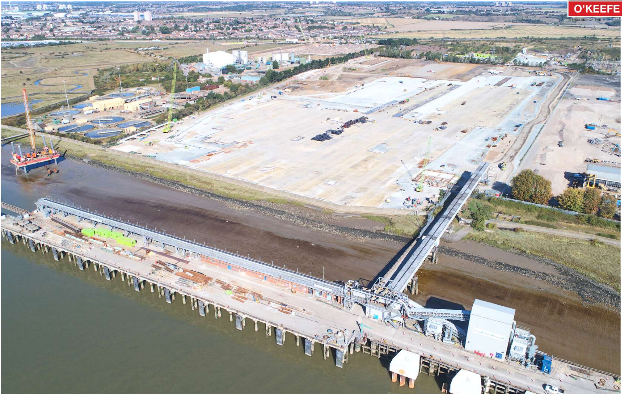
Tilbury 2 | Graham Construction | 50 Weeks | £1.2m
