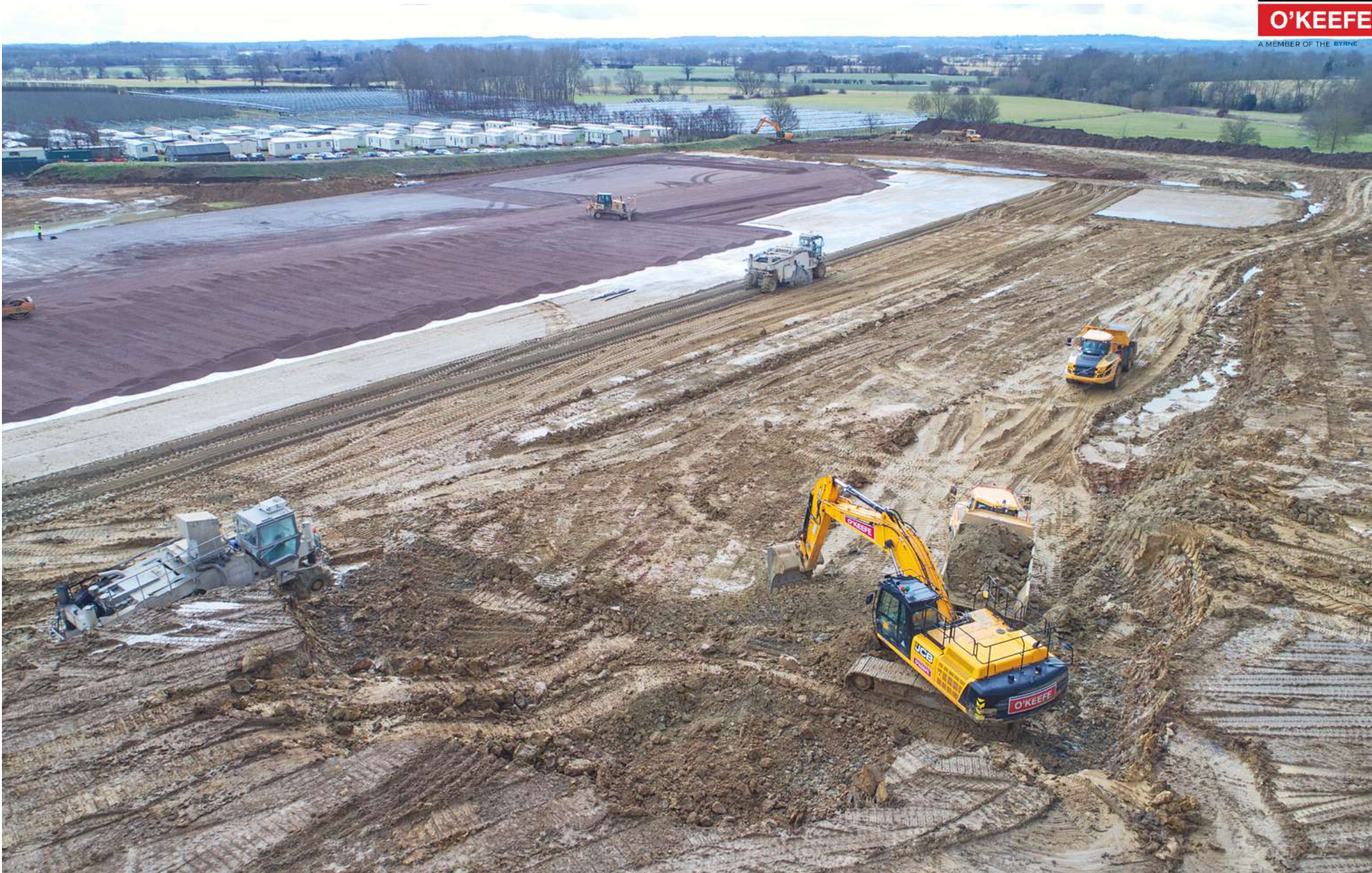
Havant Portsmouth | Civils Construction | 44 Weeks | £1.5m
